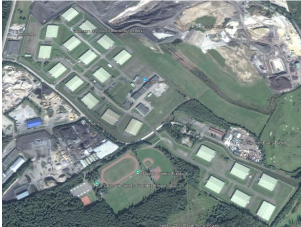
Example of a POMS site at Brunsum.
